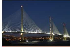
Queensferry Crossing South-Queensferry/North- Queensferry
